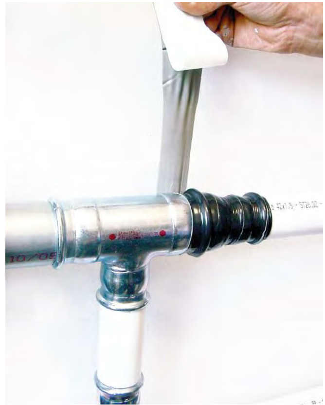
Figure 38 – Protection of the connectors with butanol adhesive tape
