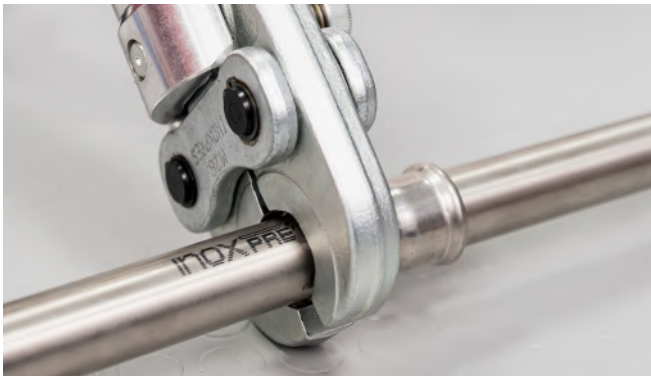
Figure 32 - Making the press connection
