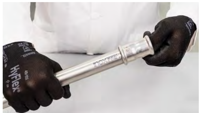
Figure 31 - Inserting pipe into the press fitting
